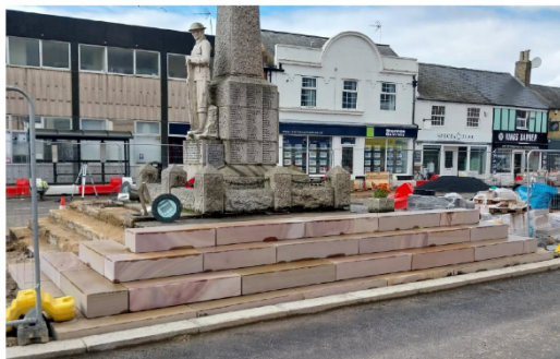
New Sand Stone Steps installation in progress
