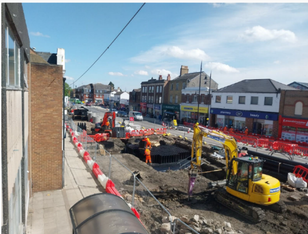
Attenuation Tank units installation in progress
